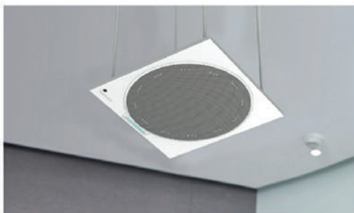
Suspending with steel rope below the ceiling.
